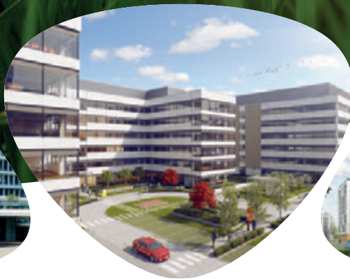
Business Garden Poznań 9 office buildings; 80,000 m 2 First phase completion 2015
