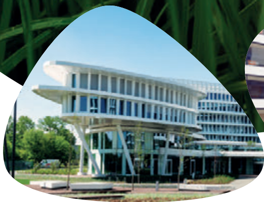
Business Garden Warszawa 7 office buildings; 90,000 m 2 Second phase completion 2016
